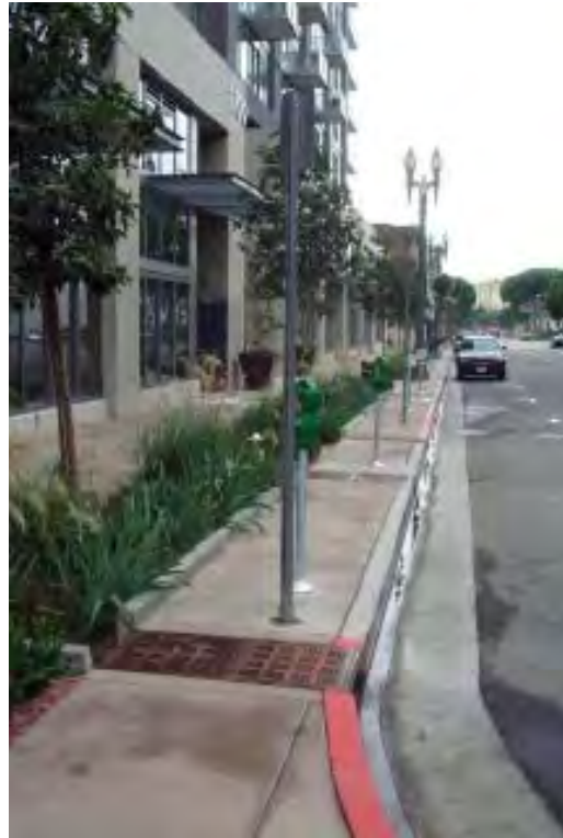
Figure 10: Bioretention cell for street/yard drainage, Los Angeles, CA. Source: Bill DePoto
