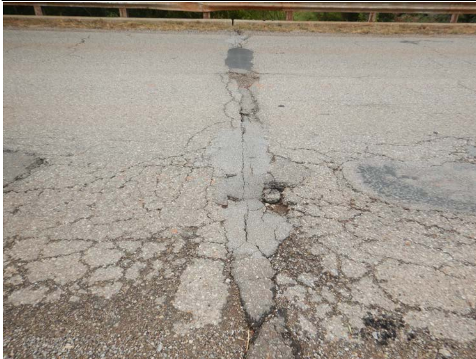
Photograph 8 - Looking east at top of deck over pier 2. Note: joints are paved over. Asphalt is cracked and spalling.
