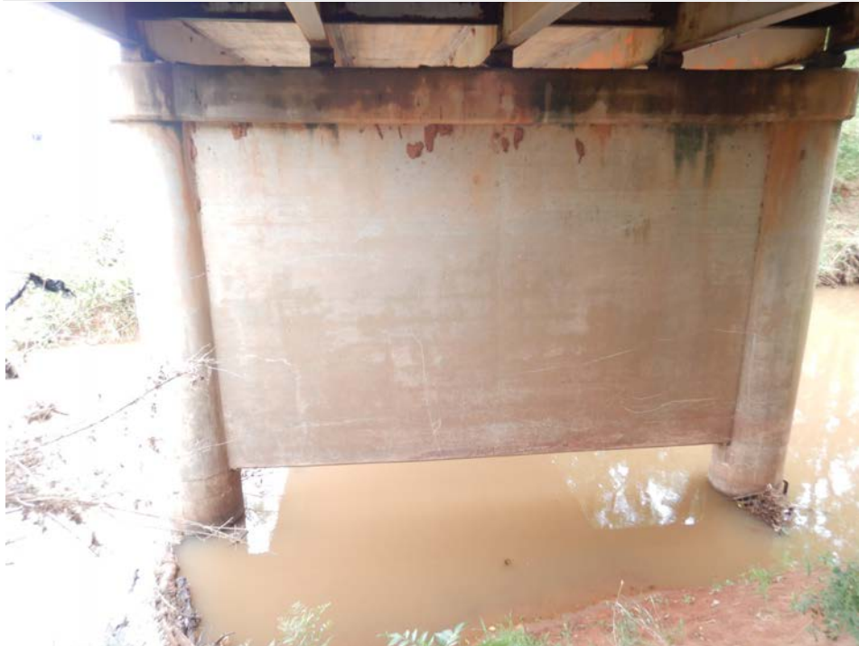
Photograph 12 - Looking north at pier 1. Note: scour exists along the south embankment. No foundations exposed at the pier.
