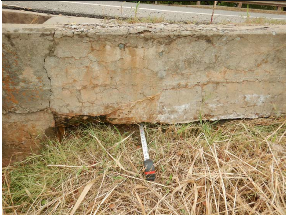
Photograph 16 - Looking east at the northwest approach roadway. Note: undermined up to 5 1/2 feet, 10 feet from the northwest corner.
