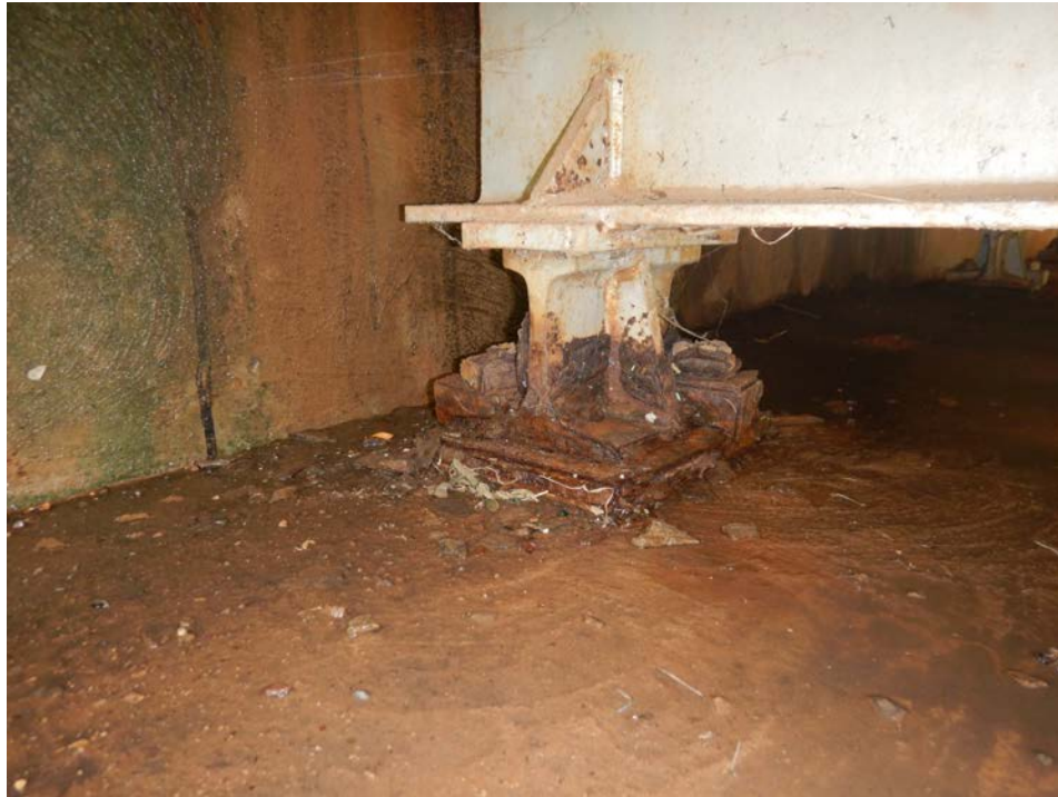
Photograph 13 - Looking west at beam 5 bearing at the south abutment. Note: pack rust and laminating corrosion exists to the bearing.
