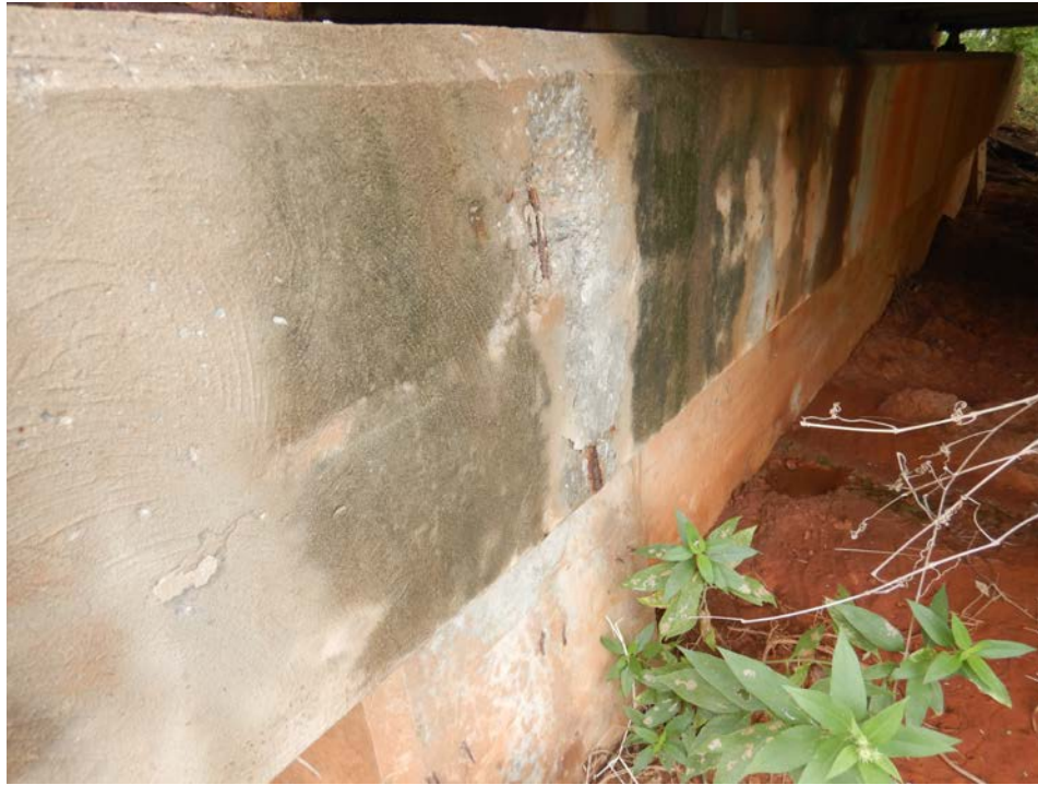
Photograph 11 - Looking northeast at the north abutment. Note: small spall with exposed reinforcing steel exists in the breastwall.
