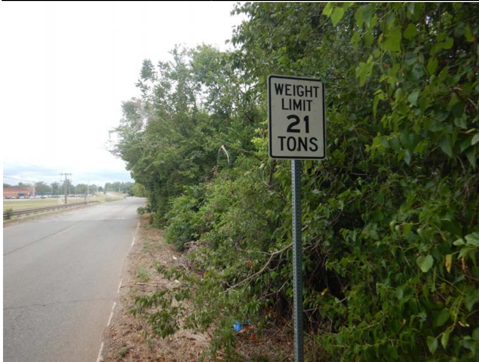
Photograph 3 - Looking north at 21 ton load posting sign in the south approach.
