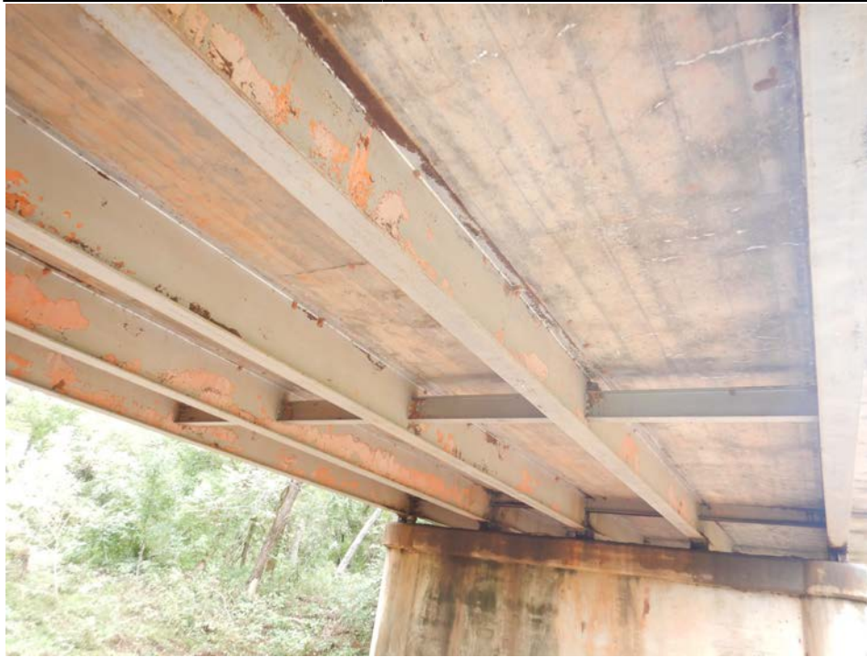
Photograph 9 - Looking south at underside span 2. Note: peeling paint and surface corrosion exists to beams.
