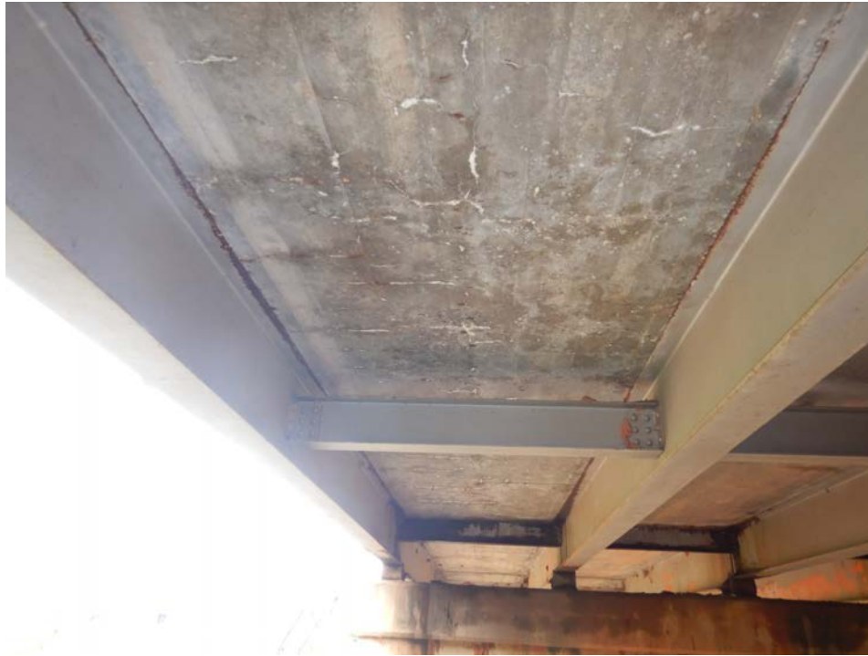
Photograph 7 - Looking north at soffit span 1. Note: transverse cracking with efflorescence common at exterior beams. Areas of cracking and spalls exist at beam ends and over intermediate diaphragms.
