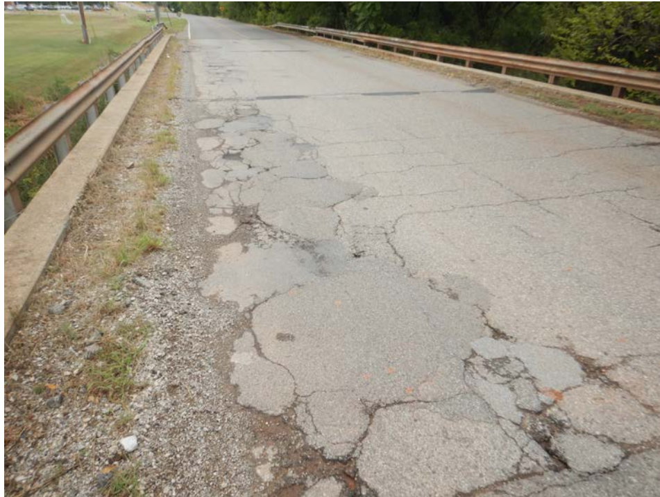
Photograph 5 - Looking north at typical bridge deck wearing surface. Note: heavy transverse cracking throughout with heavy patching in the west wheel path.
