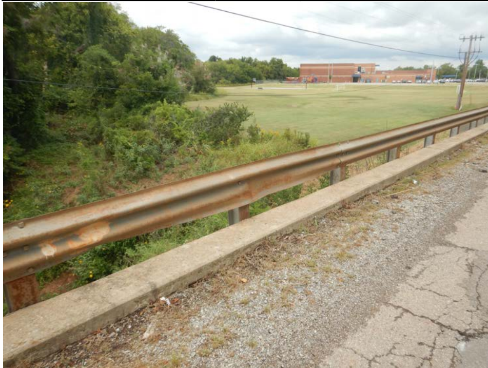
Photograph 6 - Looking northwest at span 2 west bridge rail. Note: impact damage to 5 feet.
