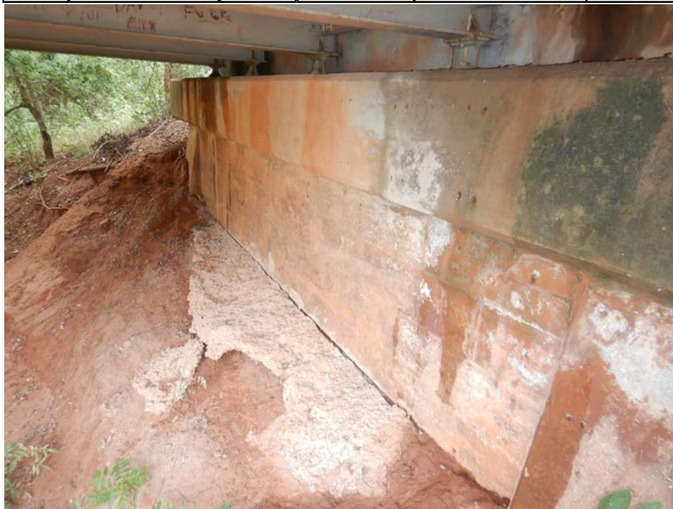
Photograph 10 - Looking east at south abutment. Note: evidence of leakage through the joint exists along the abutment.
